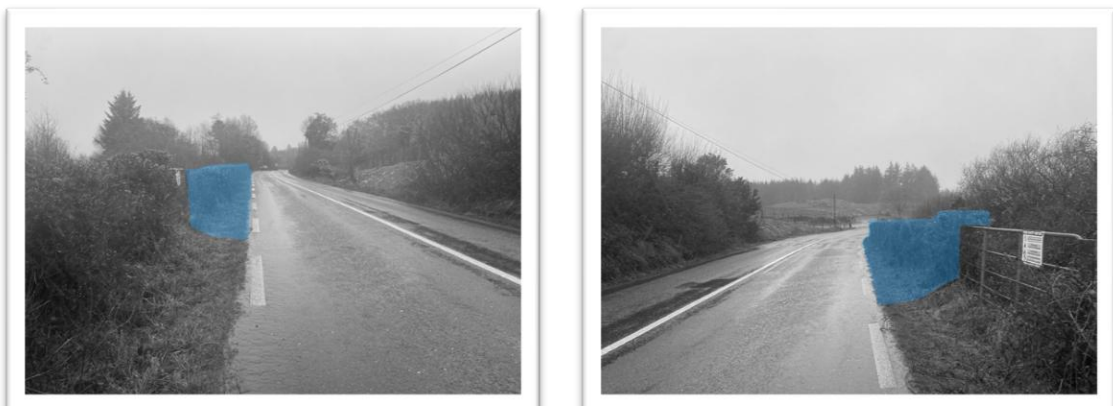
Figure 2.2 – Visibility Splays Partially Obscured in Both Directions at Site Entrance A
