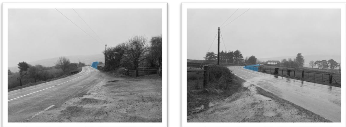
Figure 2.4 – Visibility Splays Partially Obscured in Both Directions at Site Entrance b
