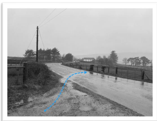
Figure 2.5 – Downhill path of storm water from Local Road into site entrance
